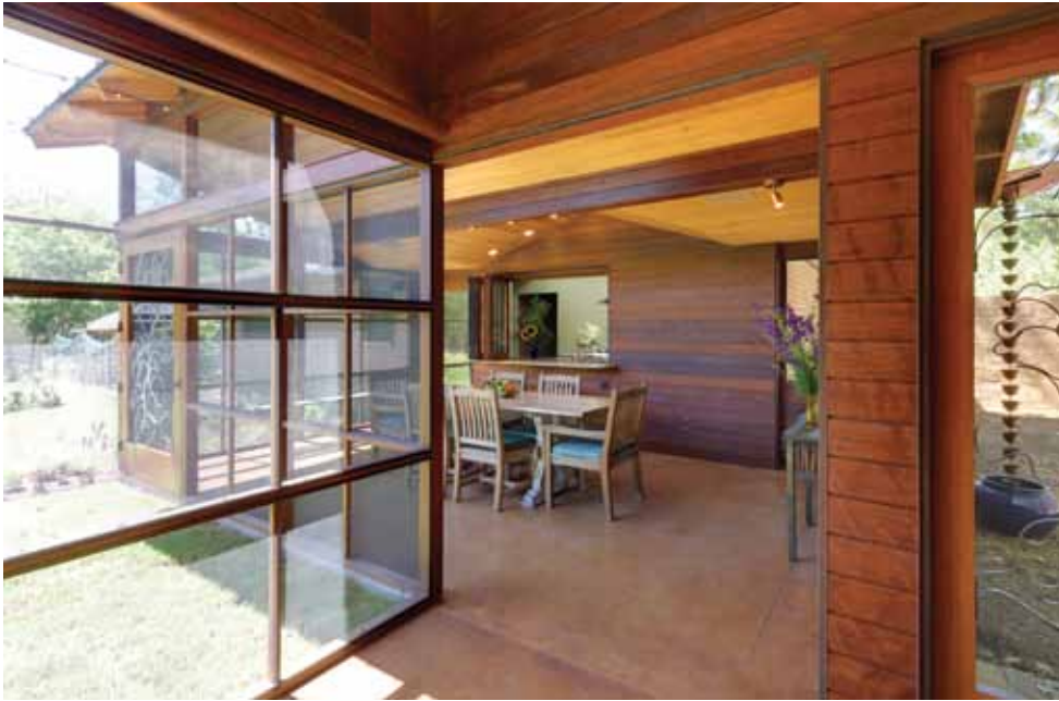
The door and screened window at right allow the southwest corner of the L-shaped addition to open to and catch the prevailing southerly, cooling breezes in summer. Note the rainwater collector and rain chain in view.
